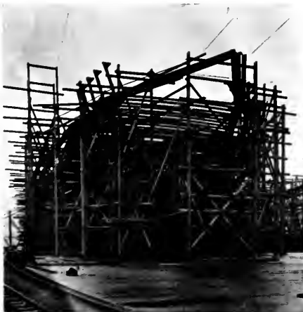
Bow view of Ship No. 1, now well under way at the yards of the Northwest Steel Company, Portland, Oregon.
